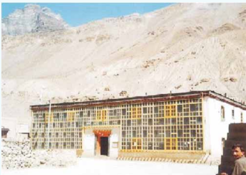
Solar Trombe Wall at Tabo Monastery Sarai
