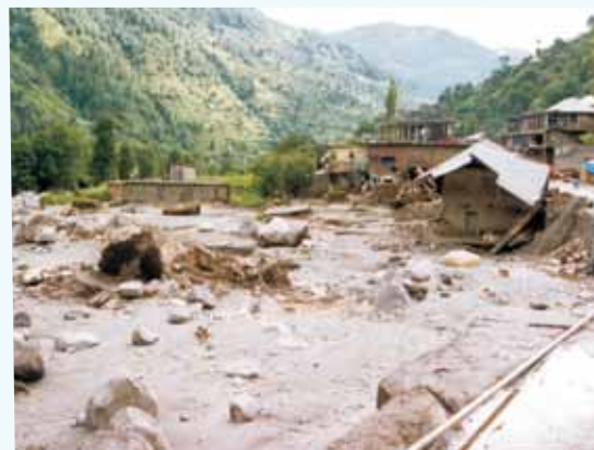
Chirgaon after cloud burst on 11 August 1997, total casualties 124
